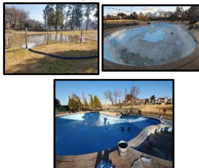
Swimming pool renovated
