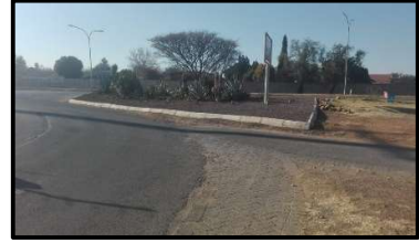
Curbs was installed at entrance to keep gravel and plants in place.
